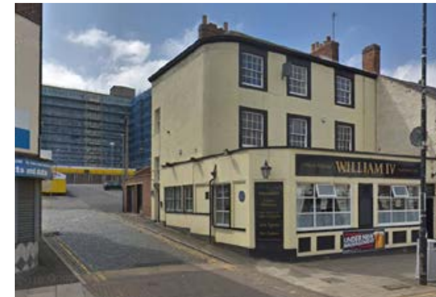
Current picture showing William IV pub on the junction Grahamsley Street
