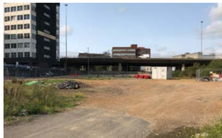
1. View looking east towards elevated Gateshead Highway
