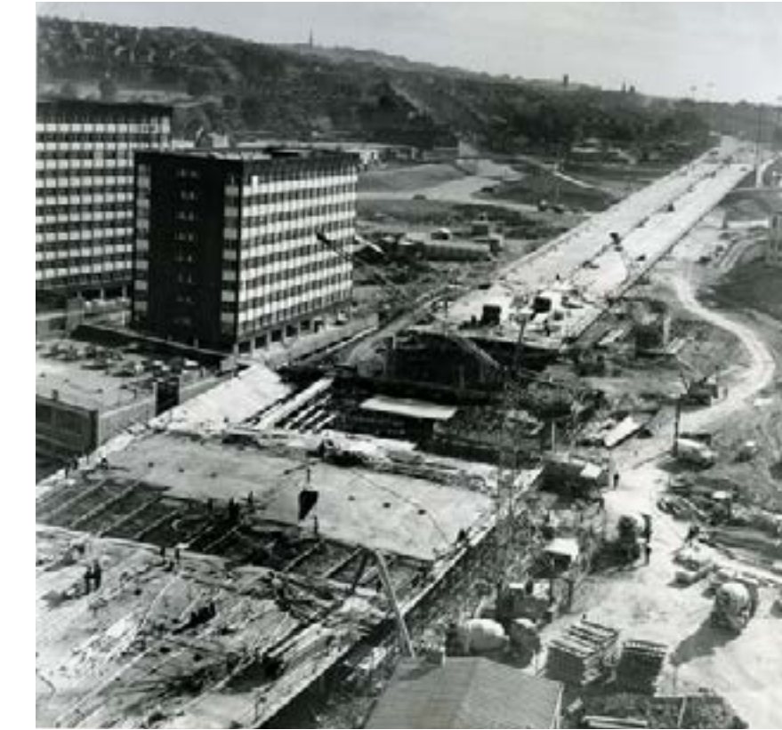
Gateshead Flyover during construction 1960's
