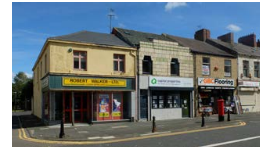
Current High Street South buildings
