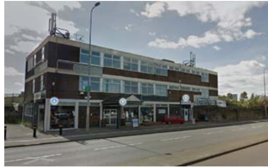
3. Exsiting building fronting Park Lane
