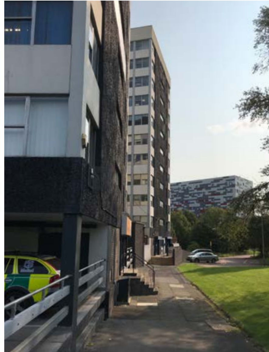
1. View of Tynegate tower blocks looking south east
