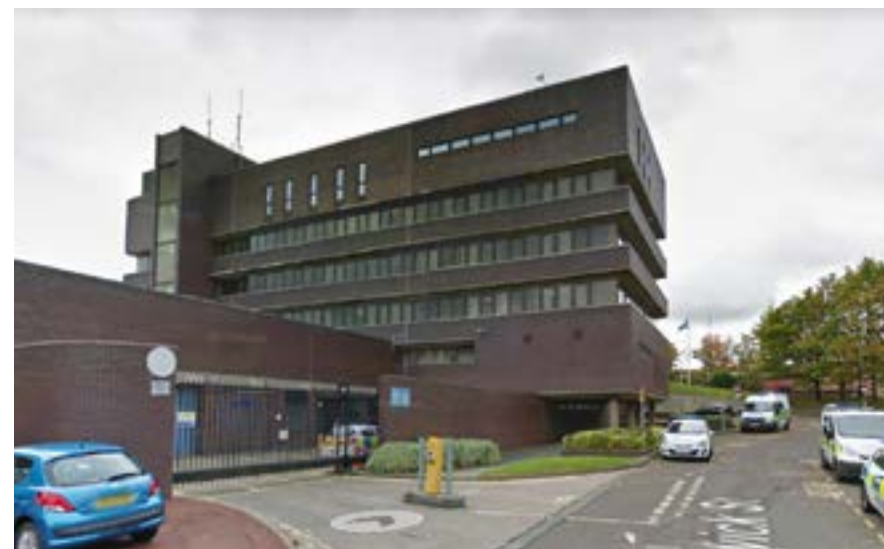
4. Police station from High West Street
